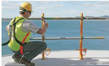
**STEP 5:** Attach Scaffold tube guardrail and midrail horizontally to the upright tube posts using standard scaffold couplers. Top Guardrail is typically set at 900mm above slab level and midrail at 500mm above slab level.
