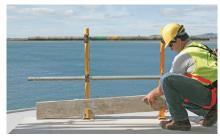
**STEP 6:** Finally, a timber toe board, typically 25mm thick, is slotted in place at the base and secured with nails or screws to the retaining bracket.
