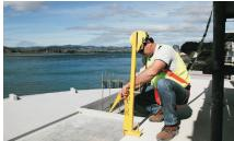
**STEP 2:** The Klamp is then positioned so that the exposed edge slots into the opening between the two parts of the Klamp. The base of the upright support rests on the top surface of the exposed edge and the slotted adjustment piece is lifted vertically until it comes into contact with the under surface of the edge.
