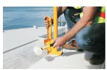
**STEP 4:** Use a mallet to drive home the wedge to tighten the Klamp against the edge. Space adjacent King Klampz at a horizontal distance of no more than 2.3m.
