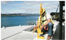
**STEP 1:** The two parts of the Klamp are separated by sliding them apart to create an opening to fit the thickness of the edge to be protected, as shown.
