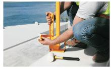
**STEP 3:** While holding the Klamp in place, insert the wedge into the adjustment slot nearest the floor.
