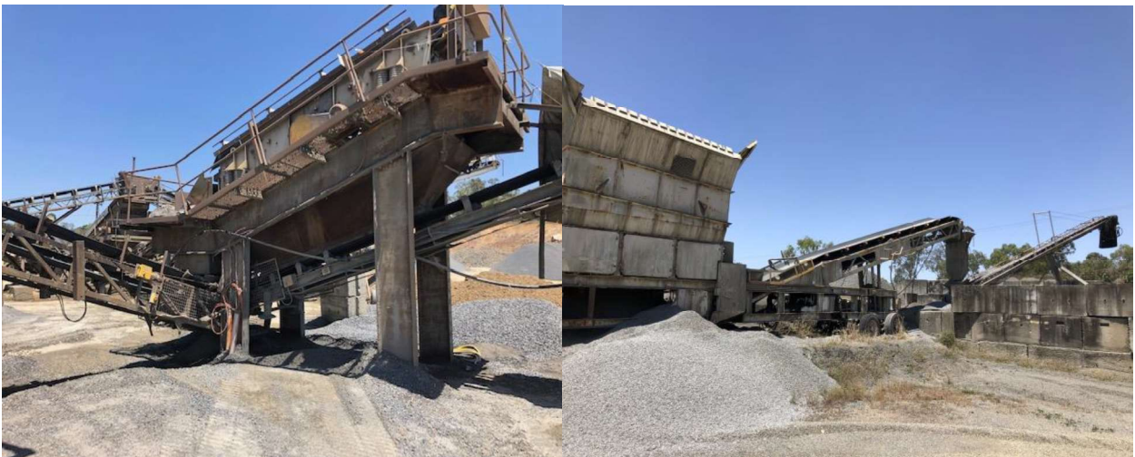
Fixed Crushing Plant
