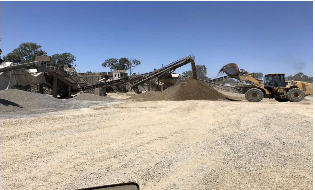
Processing Road Base
