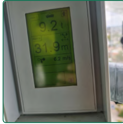
Dynamic Load Test
